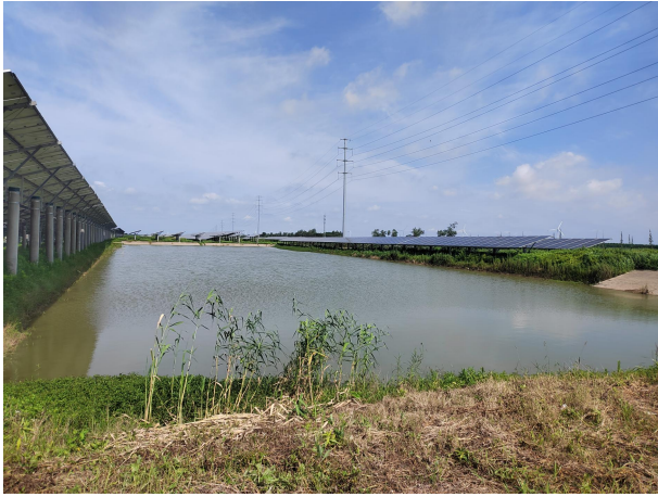
拟建“一期项目”光伏区现状
